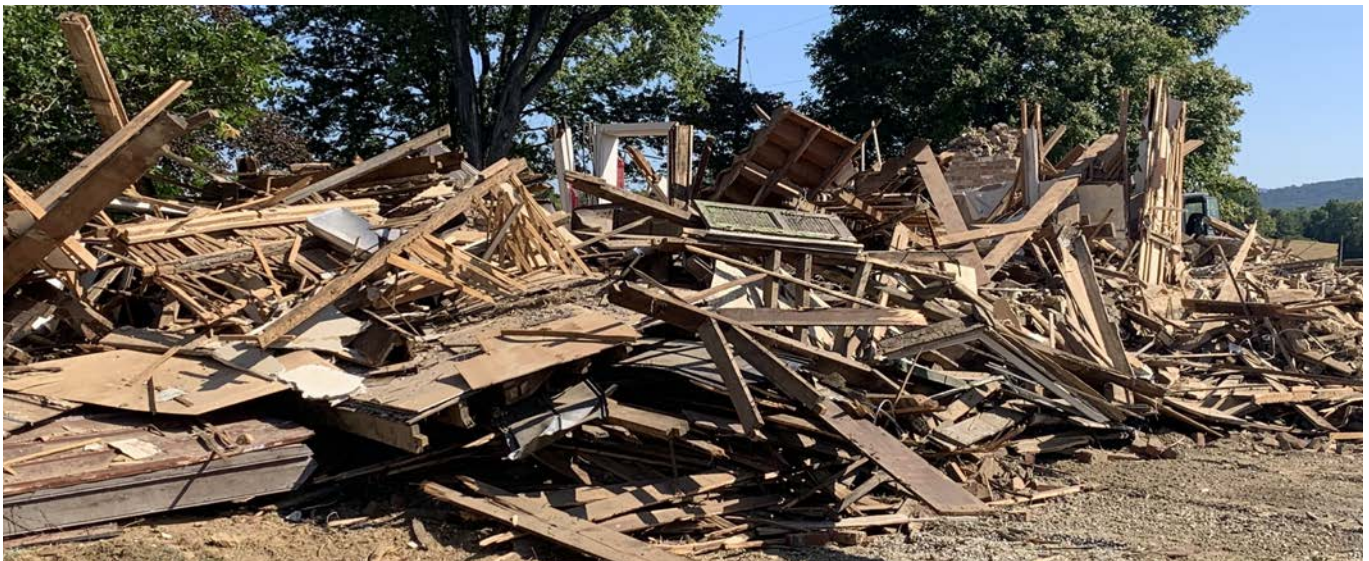
Staff Photo of Historic Property Demolition in Washington County, MD
