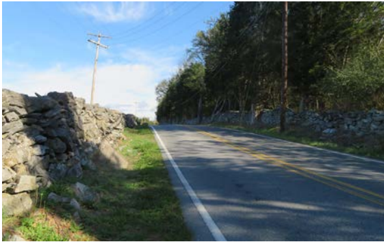
Stone Fence along Dam #4 Road, WA-II-275
