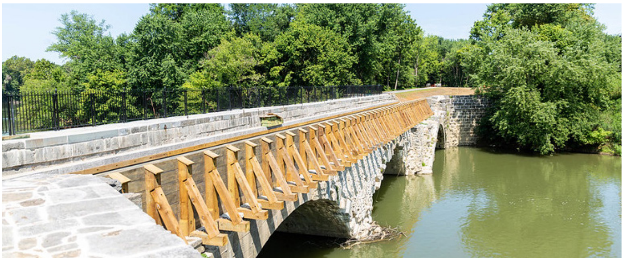
Conococheague Aqueduct, National Park Service
