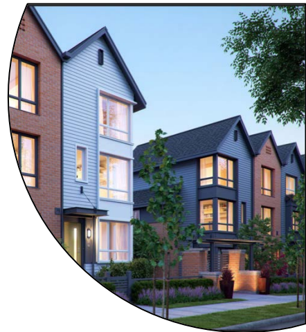
EXHIBIT 15: EXAMPLE OF MODERN TOWNHOUSES ON SMALL LOTS ARRANGED ALONG THE STREET IN A TRADITIONAL WALKABLE PATTERN.
