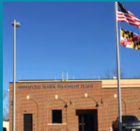
FIGURE 10-2: WATER TREATMENT PLANT
