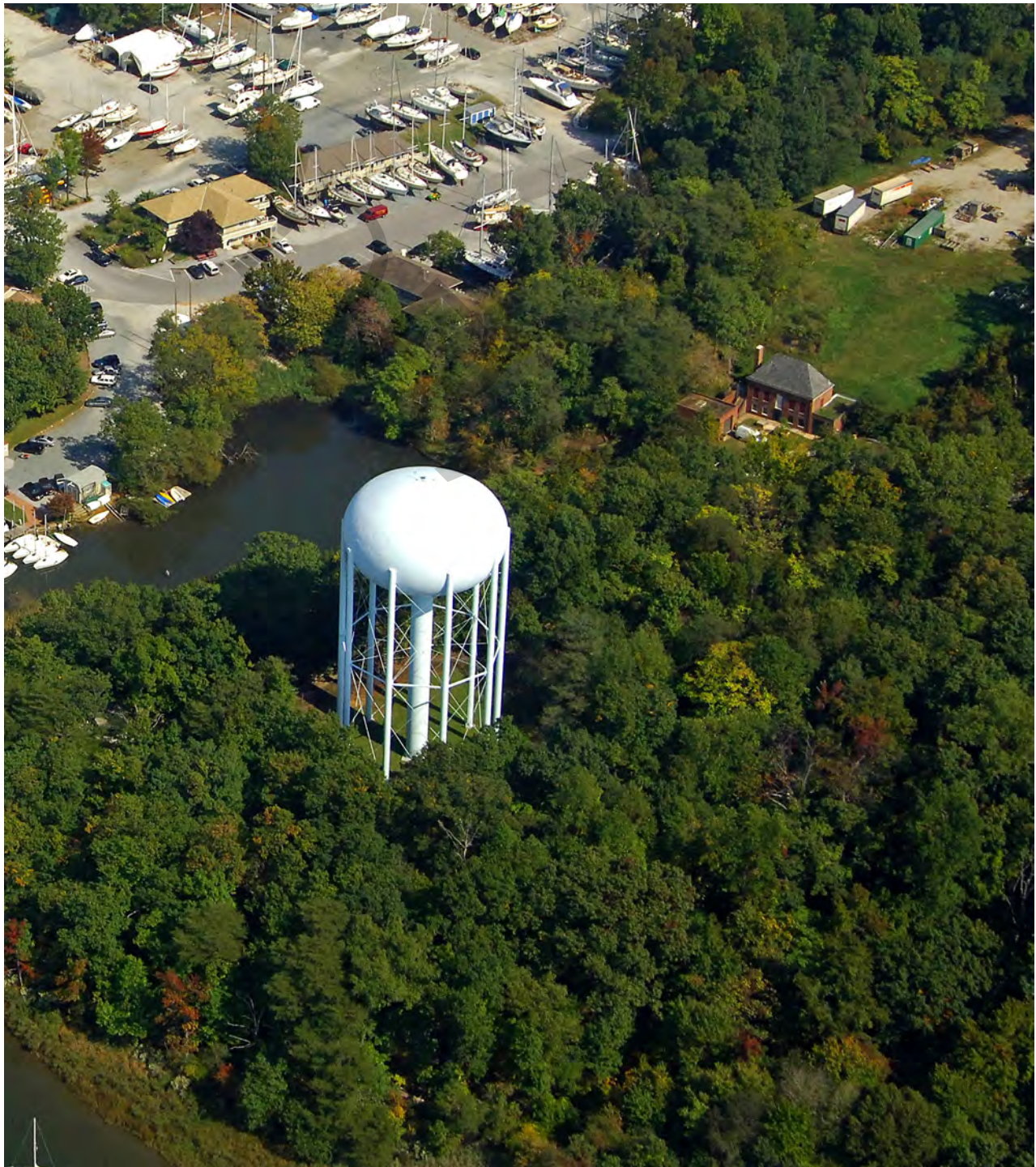
FIGURE 10-13: THE CITY'S WATER STORAGE TANK AT ELLEN O. MOYER NATURE PARK IS ONE OF FIVE ELEVATED WATER STORAGE TANKS LOCATED THROUGHOUT THE CITY.
