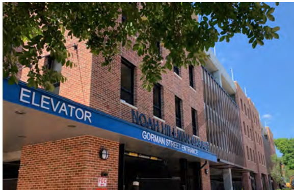
FIGURE 4-11: THE NOAH HILLMAN PARKING GARAGE IN DOWNTOWN WAS COMPLETELY REDEVELOPED IN 2022-23.
