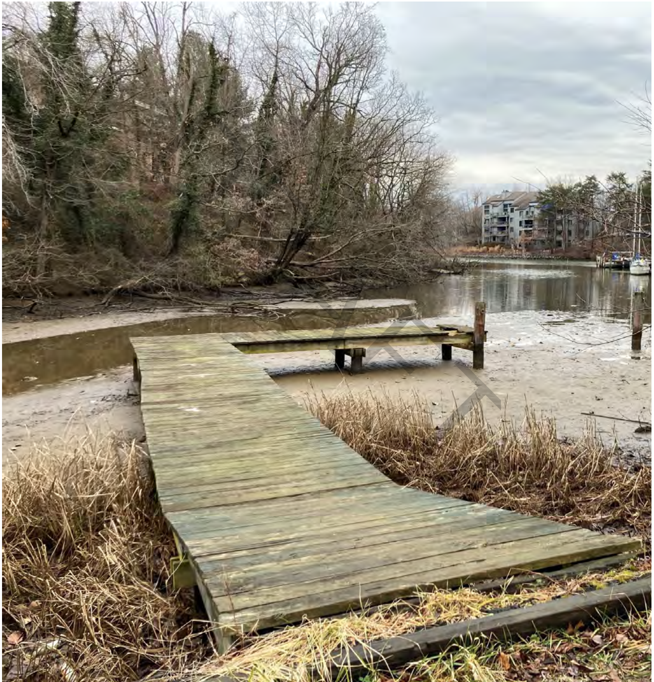
FIGURE 9-20: THE RESTORATION OF HAWKINS COVE IS A CITY PRIORITY BECAUSE IT WILL ADDRESS MULTIPLE CITY ENVIRONMENTAL GOALS INCLUDING WATER QUALITY IMPROVEMENT, HABITAT ENHANCEMENT, AND WATER ACCESS.
