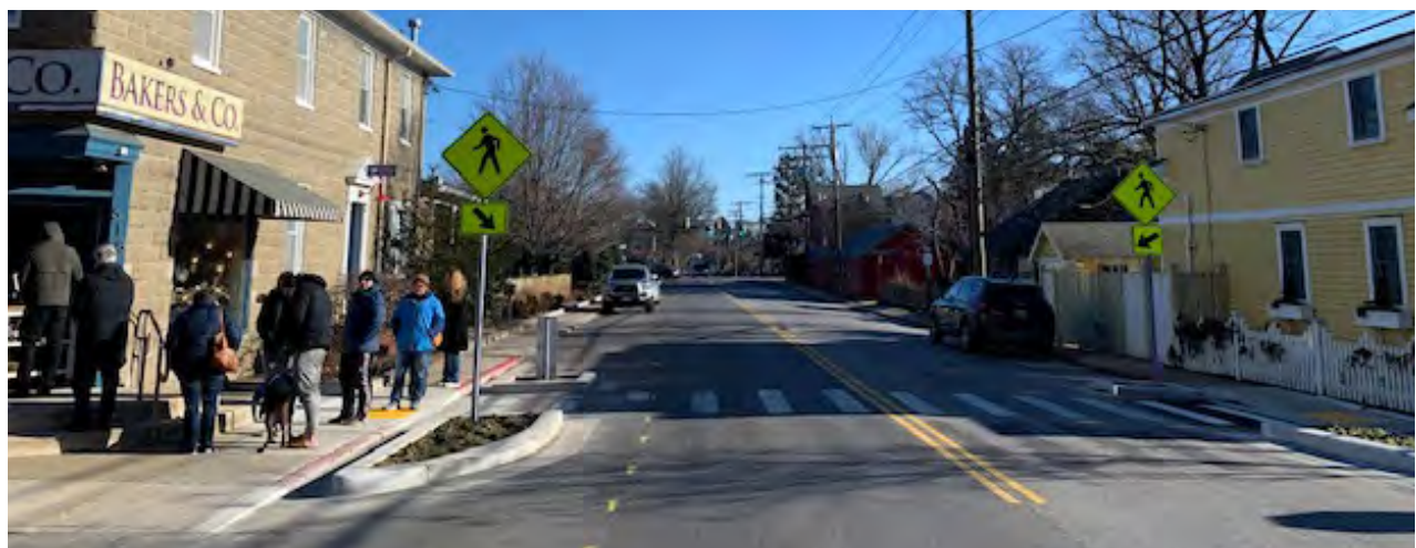
FIGURE 6-15: THIS RECENT INTERSECTION IMPROVEMENT ON CHESAPEAKE AVENUE SHORTENS THE CROSSING DISTANCE FOR PEDESTRIANS, CALMS VEHICULAR TRAFFIC, AND ADDS PLANTINGS.
