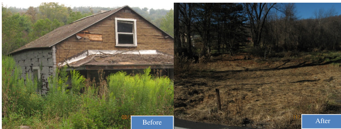
Figure 4-1: Unsafe Structure Removal
