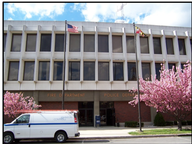
Fire & Police Department Headquarters
