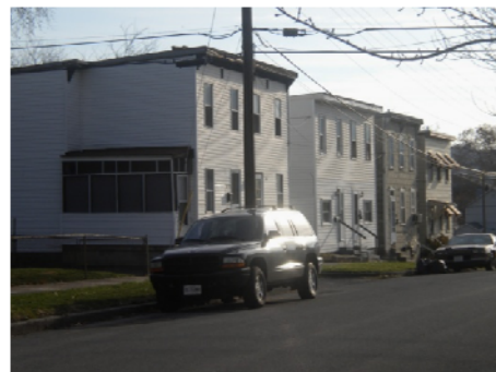
Typical Railroad Flat Homes
