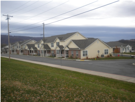
The New Gateway Townhomes Project
