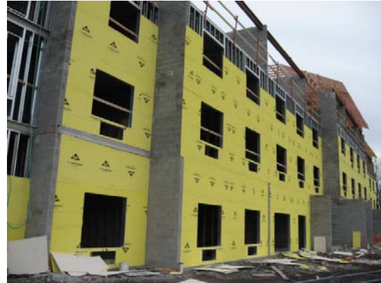
New Hotel Construction in Canal Place
