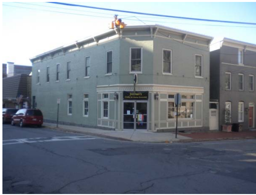
Commercial Rehab at Decatur St. & Baltimore Ave.
