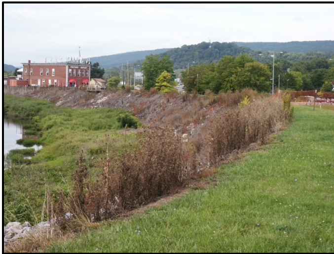
Proposed Riverwalk Location along the levee
