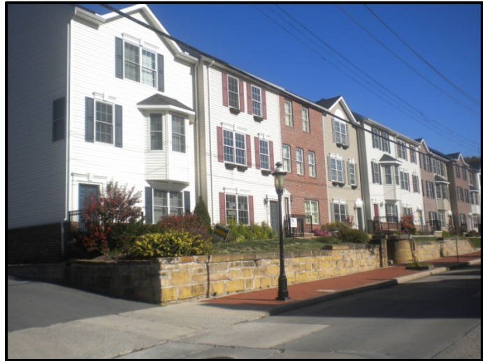
Townhome Redevelopment on Decatur Street
