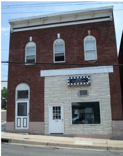
402 Virginia Ave. Before Façade Restoration
