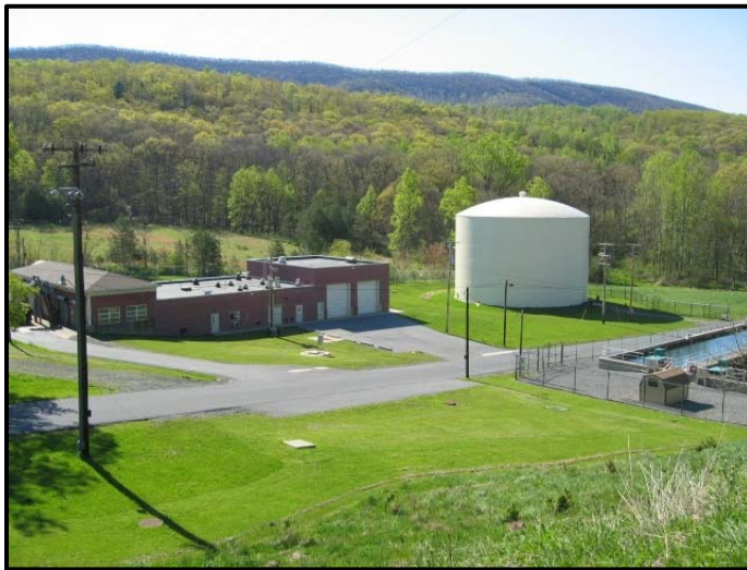
Cumberland's Water Filtration Plant
