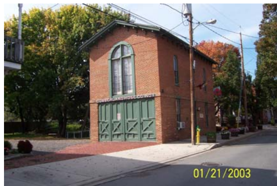
Canada Hose Company Building - N. Mechanic Street
