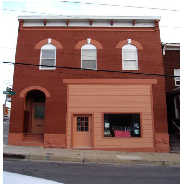
402 Virginia Ave. After Façade Restoration
