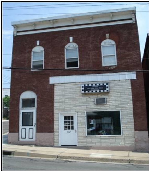
Virginia Ave. Building before rehab work
