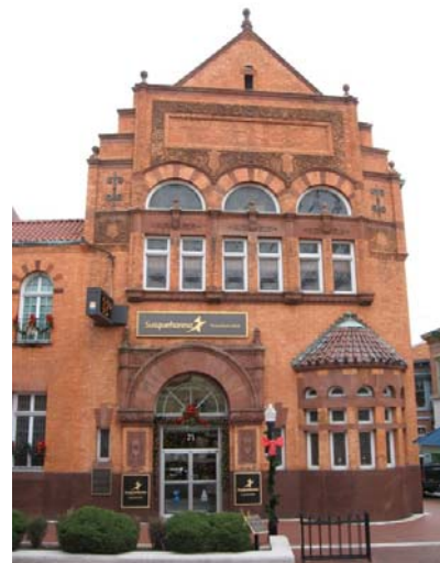
Historic Commercial Architecture on the Downtown Mall
