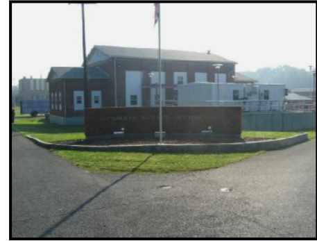
The Sewer Treatment Plant
