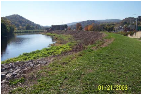
North Branch Potomac River Levee
