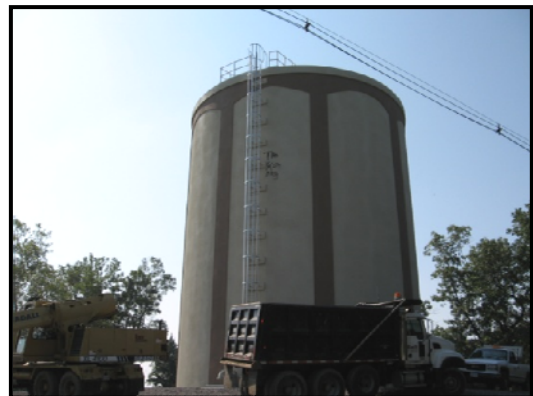
Fort Hill Storage Tank
