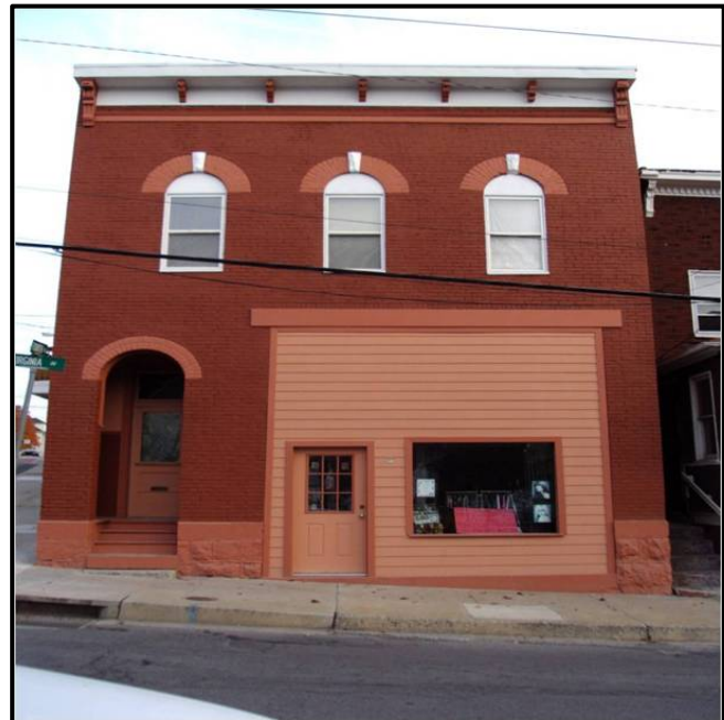
Virginia Ave. Building after rehab work
