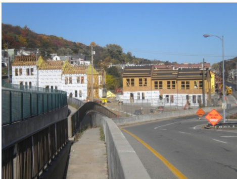
Banneker Gardens under Construction
