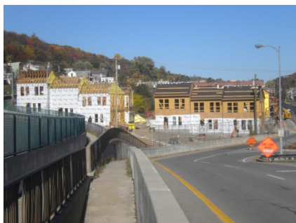
Banneker Gardens Construction
