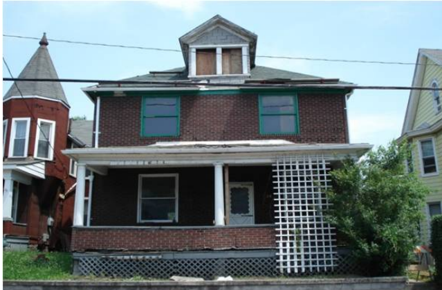
Chapel Hill Home before Facade Revitalization
