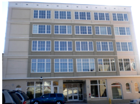
The Vista Tower Rehab Project
