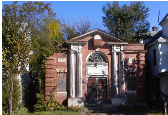
The old “Hillsboro Bank Building” has been purchased by the Town and is presently being restored as a museum and tourism information center.
