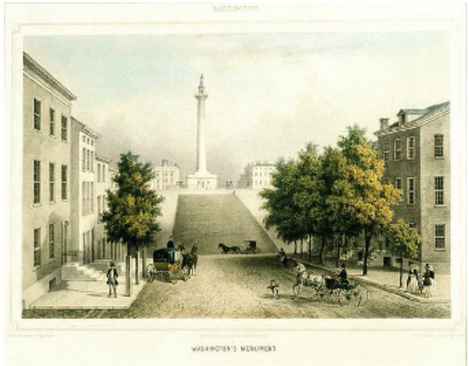
An 1848 image of the Washington Monument from Charles and Hamilton streets. The squares were first laid out as simple lawns.
