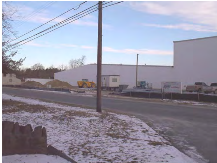
New Maryland Plastics Facility under Construction
