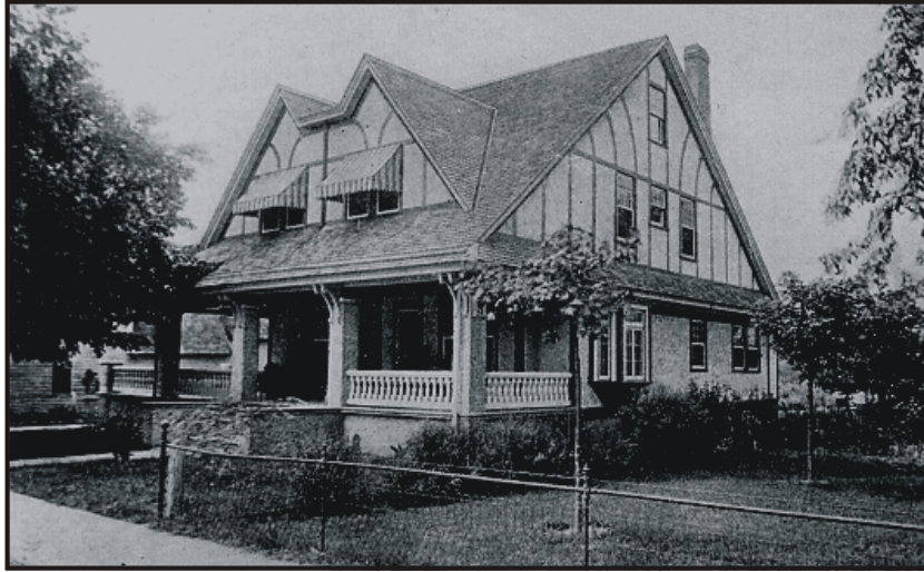
Carroll Residence on East Central Avenue
