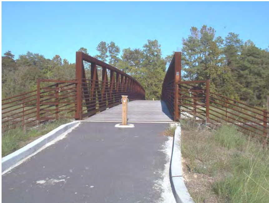
The Pedestrian Bridge on the River walk
