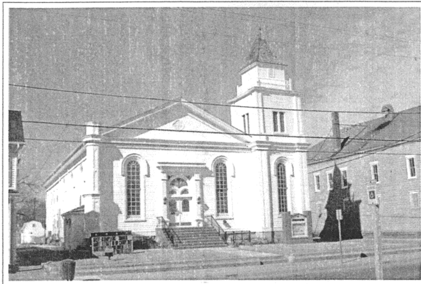
Union Methodist Church (on the west side of South Main Street) just completed a major renovation.
