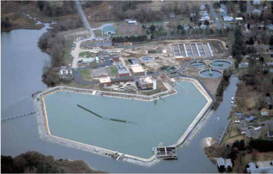
Cambridge wastewater treatment plant.
