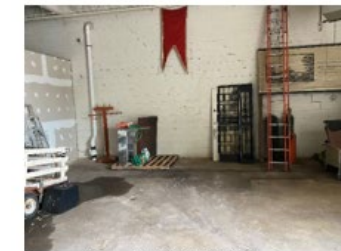
Photograph 5. SECONDARY SYSTEM – Fan Fan should be running, with minimal noise there should be no loose connections
