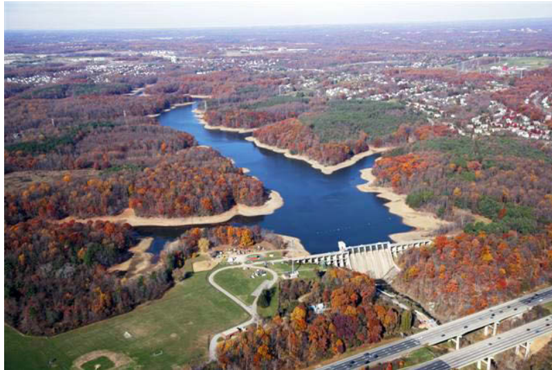
Washington Suburban Sanitary Commission's Triadelphia Dam, Prince George's and Howard Counties
