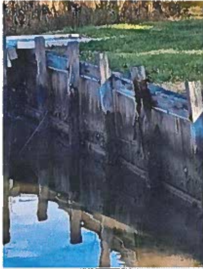
Bulkhead to be replaced with a Living Shoreline
