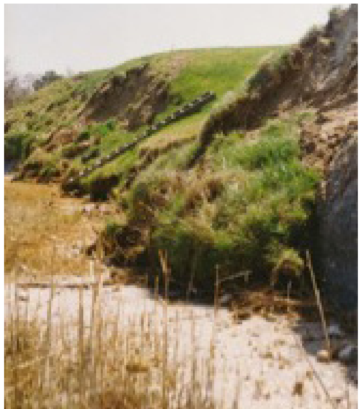
After (Soil Erosion)
