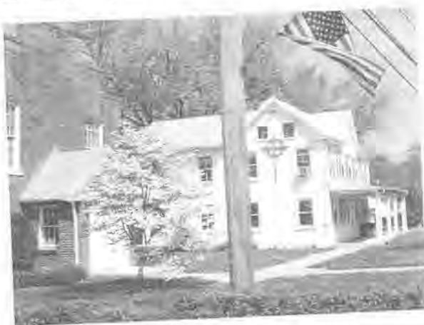
Whites Ferry Road building (shown) is at risk of erosion.
