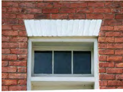
Jack arch framed by brick
