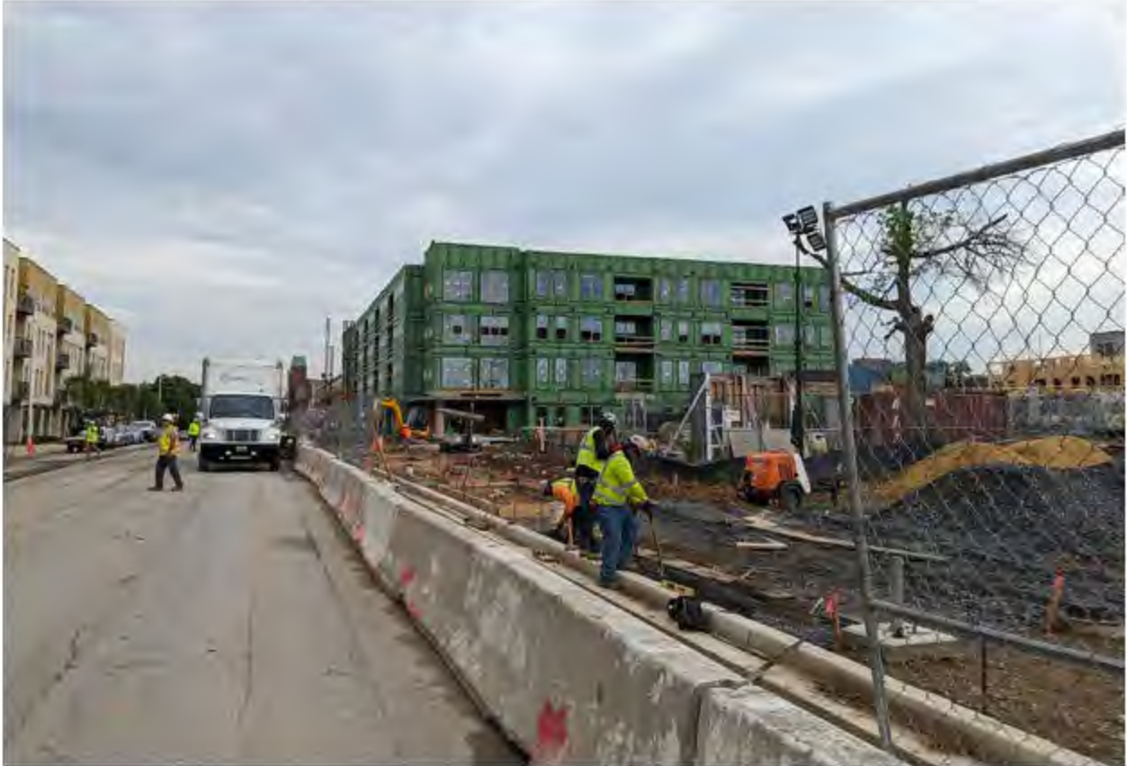
Roadway improvements related to Perkins Somerset Oldtown redevelopment.
