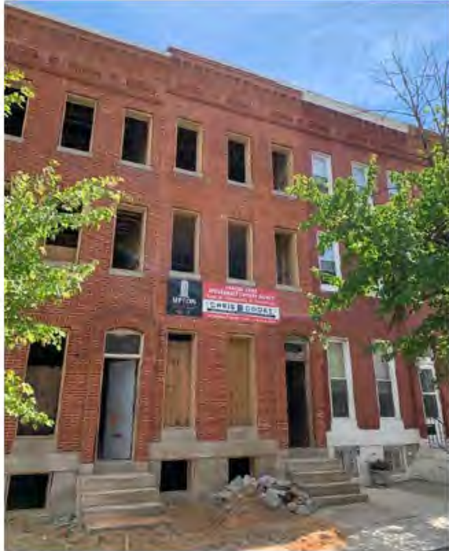
Renovation underway in Upton.
