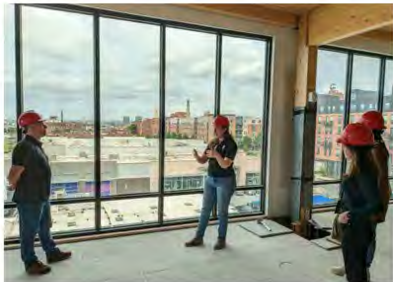
A building under construction near many newly constructed multi-family buildings.
