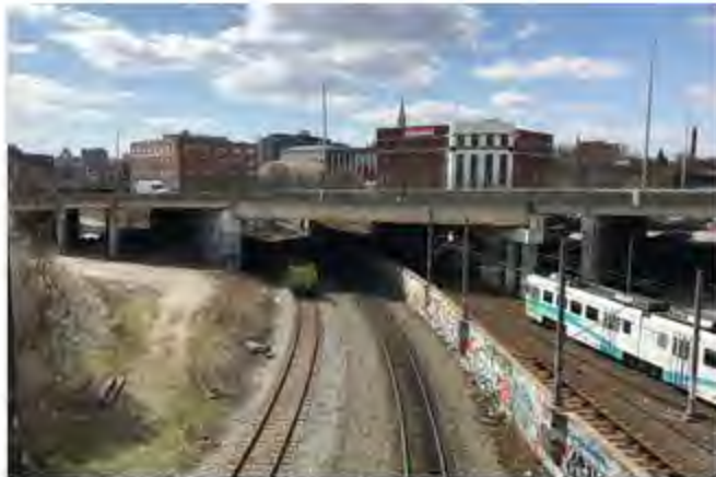
MTA Light RailLink under Interstate 83.
