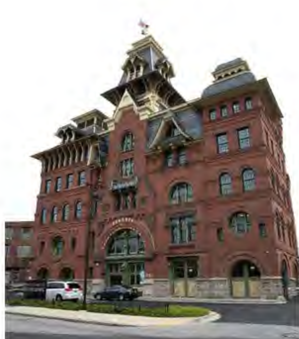
The American Brewery building.
