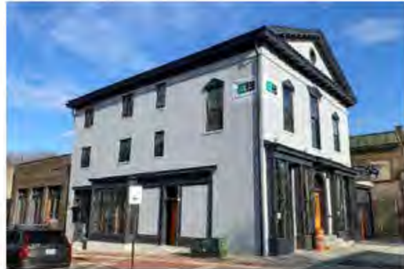
Recently renovated Waverly Town Hall, a Baltimore City Landmark.
