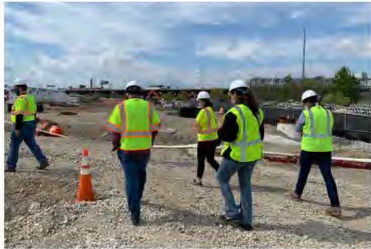
A construction site in South Baltimore.
