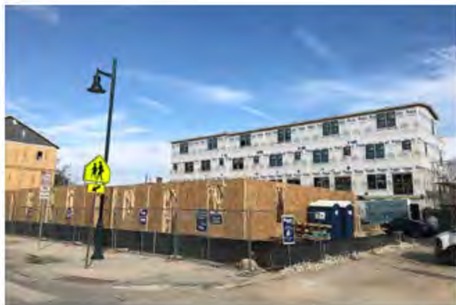
Construction of new residential housing.
