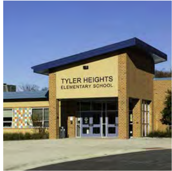
FIGURE 4-10: TYLER HEIGHTS ELEMENTARY WAS FULLY RENOVATED IN 2022 BY ANNE ARUNDEL COUNTY PUBLIC SCHOOLS AND IS A HUB FOR THE COMMUNITY.
