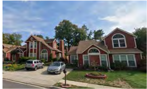
FIGURE 5-5: SINGLE FAMILY DETACHED HOMES NEAR EDGEWOOD ROAD
