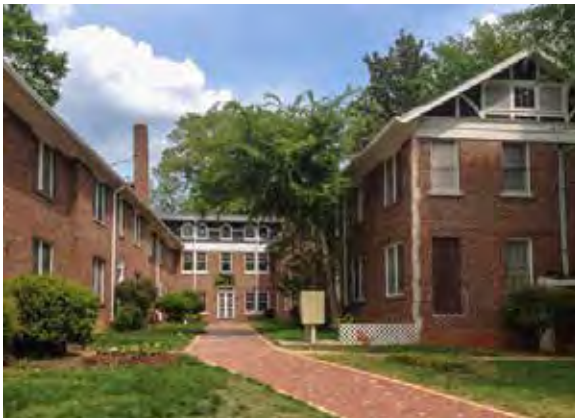
FIGURE 5-33: COURTYARD BUILDING: A DETACHED BUILDING TYPICALLY LARGER BUT NOT NECESSARILY TALLER THAN A SINGLE FAMILY HOUSE, CONTAINING MULTIPLE DWELLING UNITS SITUATED AROUND A SHARED COURTYARD WITH A SHARED BUILDING ENTRANCE.
