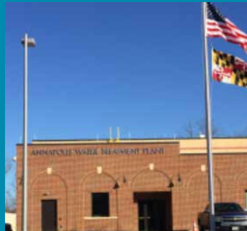
FIGURE 10-2: WATER TREATMENT PLANT
