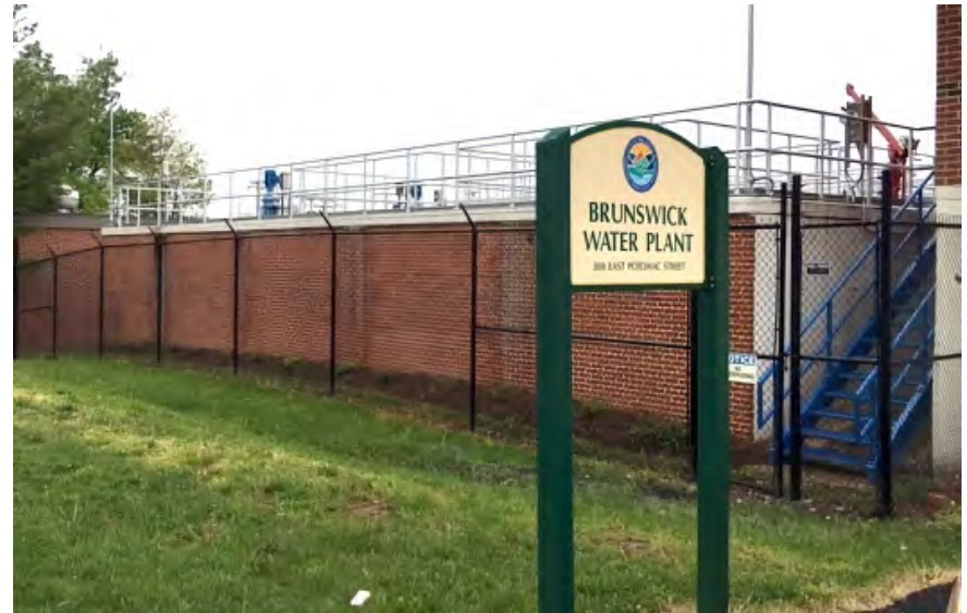
Located at 300 East Potomac Street just southwest of Downtown Brunswick, the Brunswick Water Treatment Plant withdraws and processes water from the Potomac River.
