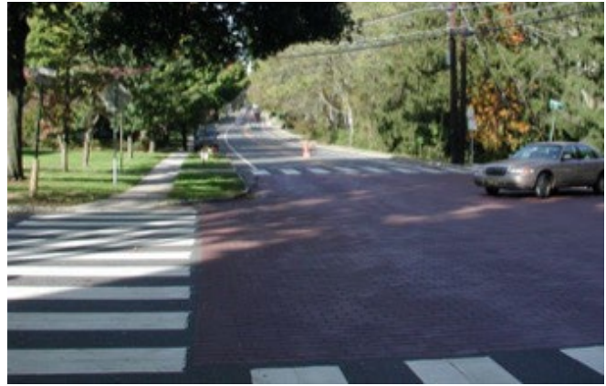
Figure 20 - High visibility "Continental" type crosswalks can be striped to reduce tire track wear through the gaps and are recommended for gateway and transition areas to increase pedestrian safety
