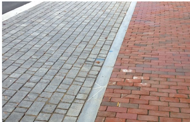
Figure 19 - Within the core area of town, the parking areas should be paved with permeable pavers (granite cobbles or textured concrete pavers with similar character to cobbles with engineered subbase designed to encourage infiltration for stormwater)
