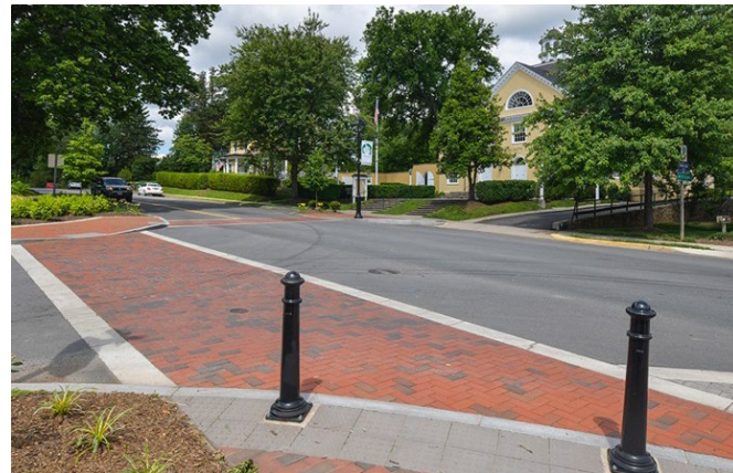
Figure 21 - Within historically sensitive areas associated with the Primary Historic Resources, brick crosswalks can be installed and striped using a concrete band (need to contain the bricks) tinted white to increase visibility.
