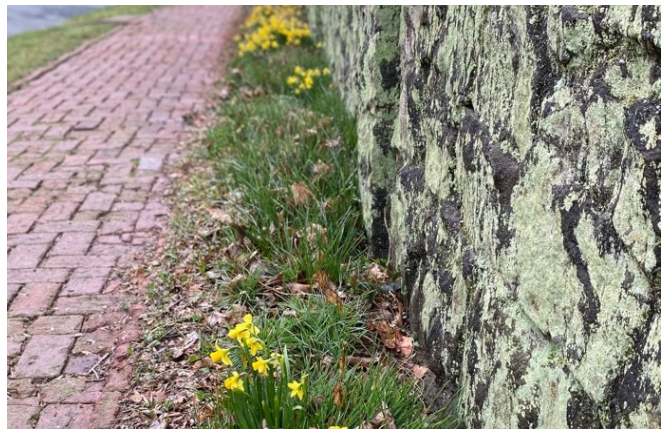
Figure 18 - Brick sidewalks with planting strips are recommended for transition areas and core areas within the Town
