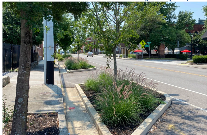
Figure 40 - Vegetated buffer strips can store and filter stormwater
