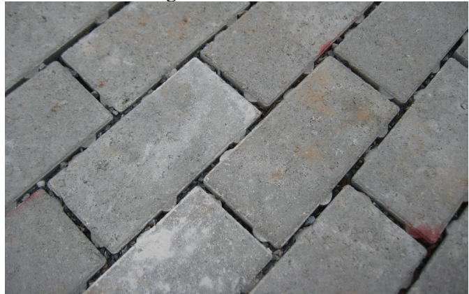
Figure 39 - Permeable pavers allow stormwater to be filtered, stored, and or redirected to a stormwater management facility
