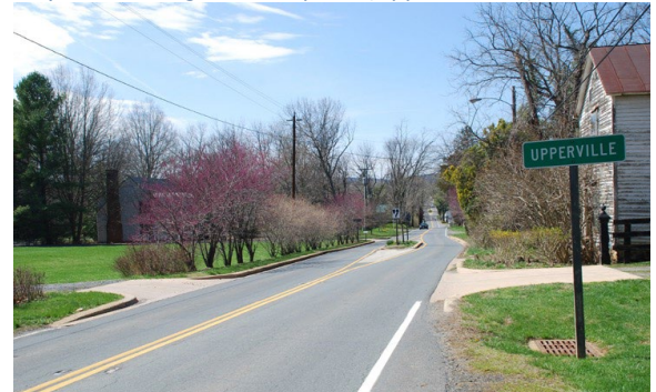
Figure 15 - At the southern end of town utilize a narrow splitter island as a traffic calming measure coordinated with the location of a proposed crosswalk (Upperville, VA)
