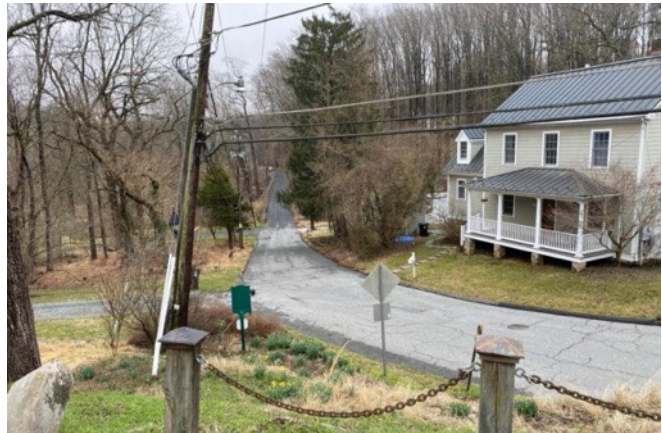
Figure 35 - Existing extruded asphalt curbs should be replaced with concrete curb and gutter in the gateway area (and with granite curbs in transition areas and in town). A flush curb should be installed in advance of the gateway to alert drivers that they are entering a settled place.
