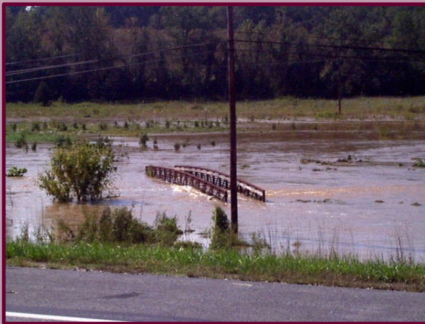
Little Pipe Creek Park Bridge
