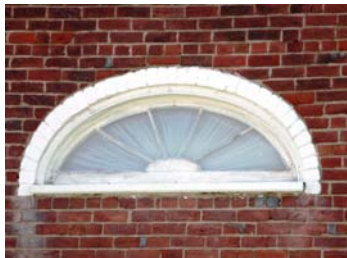
Eye-brow, lancet windows and fan lights
