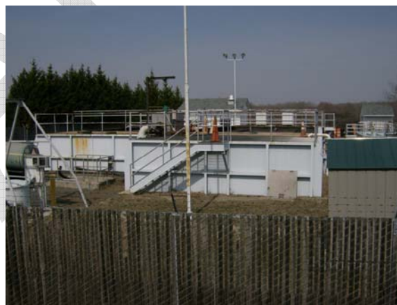
The Town's wastewater treatment plant is located along the Nanticoke River on the north side of town. The plant is 35 years old and will likely need upgrading to keep pace with new environmental restrictions.
