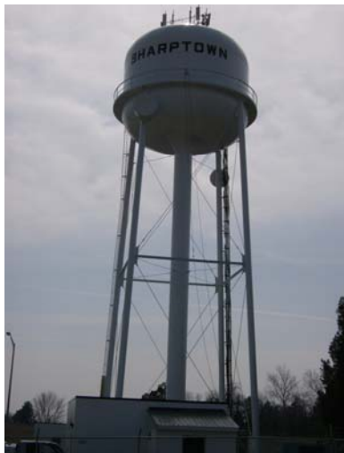
The Sharptown elevated water tower, shown here, was built in 1990 and has a 200,000 gallon capacity.
