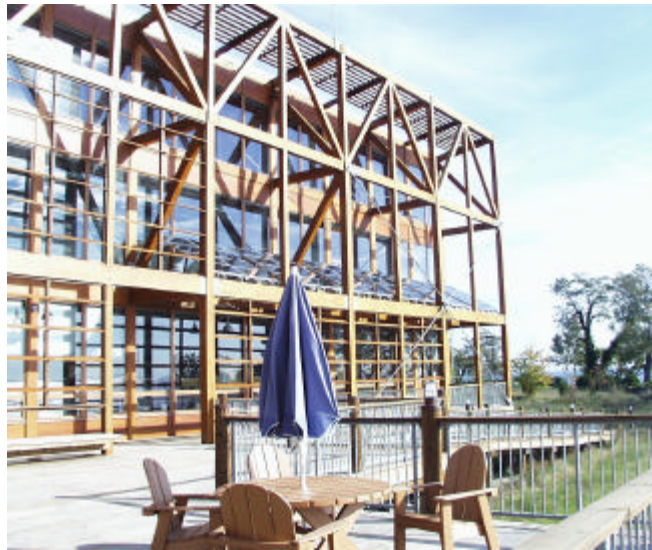
Figure 17 The Chesapeake Bay Foundation's Philip Merrill Environmental Center, in Annapolis, Maryland, was the first building to receive a LEED Platinum Rating from the U.S. Green Building Council.
