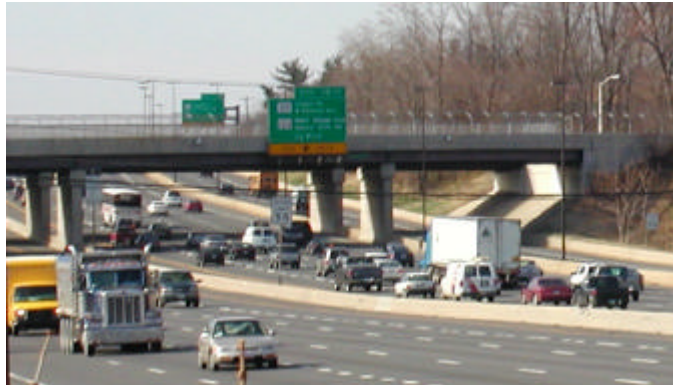
Figure 14 On-road mobile sources, such as the traffic on Interstate 270, account for 34 percent of nitrogen oxide emissions (NOx) and 35 percent of volatile organic compounds (VOCs) emissions in Montgomery County.
