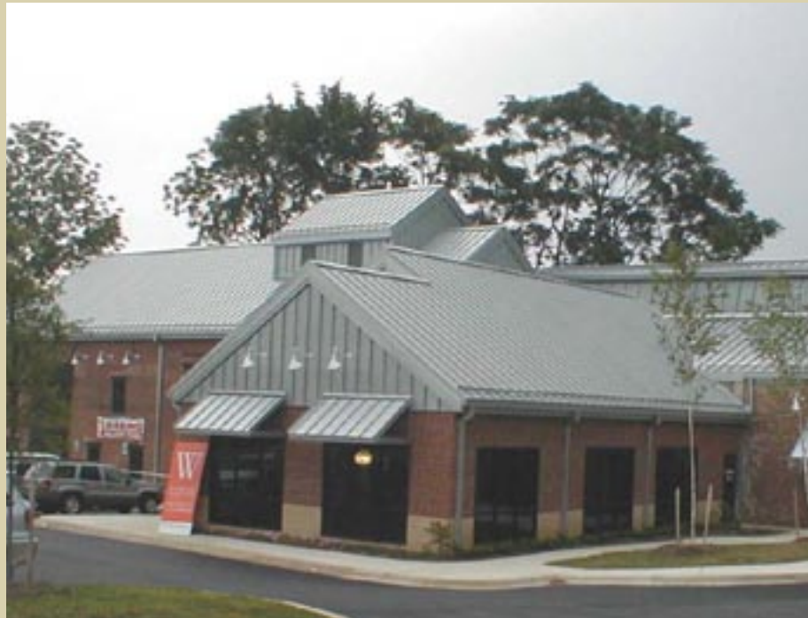
The newly-restored Thomas Cannery Building increased available commercial space while preserving a piece of Olde Towne's past.
