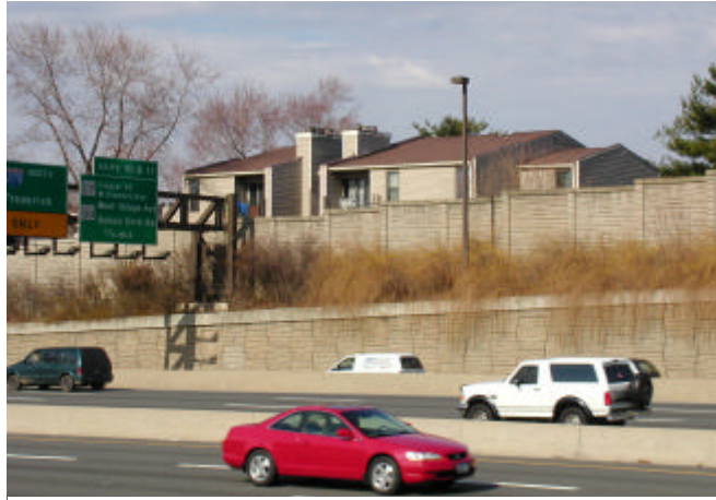
Figure 19 Automobile and truck traffic along major roadways is a significant source of noise pollution. Noise walls, as illustrated above, are constructed to mitigate noise in severe circumstances.
