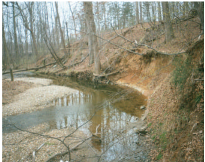
Figure 6 Steep slopes and erodible soils hydraulically adjacent to streams, as indicated in the above photo of the Muddy Branch, illustrate why these are sensitive areas in need of special protection.
