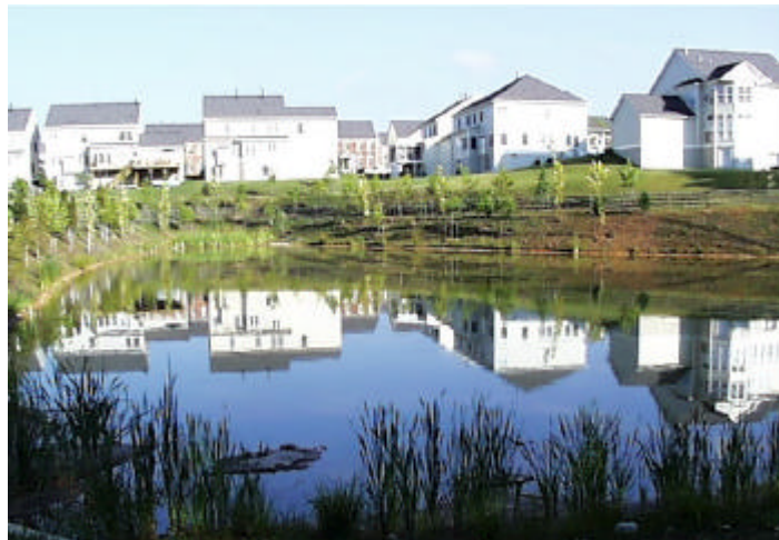
Figure 5 The stormwater management pond in Quince Orchard Park treats runoff, provides wetland habitat, and serves as a community amenity.
