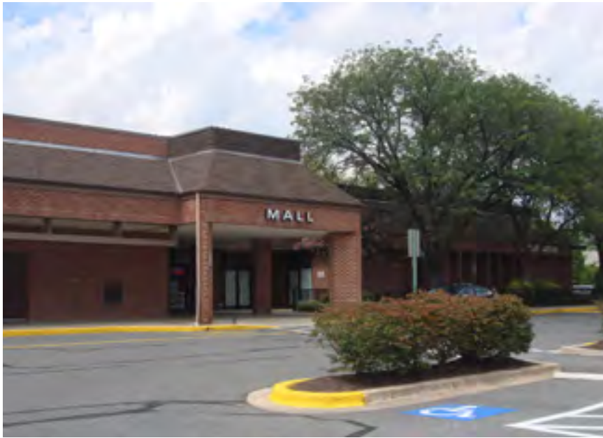
Front entrance of the former Rockshire Shopping Center
