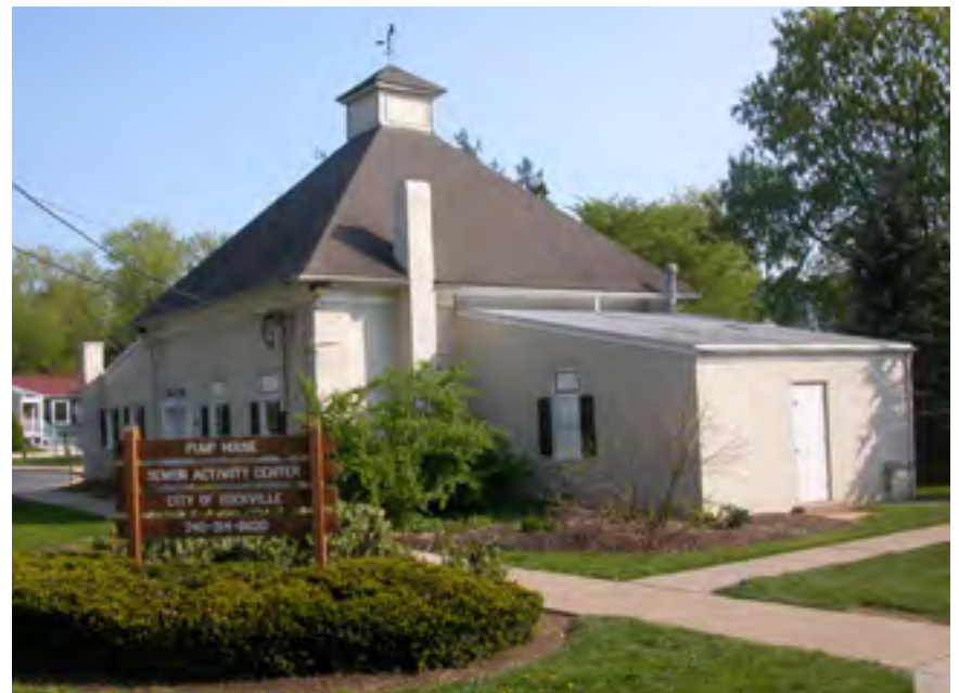
The Pump House at 401 S. Horners Lane is an example of adaptive reuse of a locally designated historic property, owned by the City of Rockville and retrofitted from a water pump house to an activity center with meeting room used primarily by the East Rockville community.
