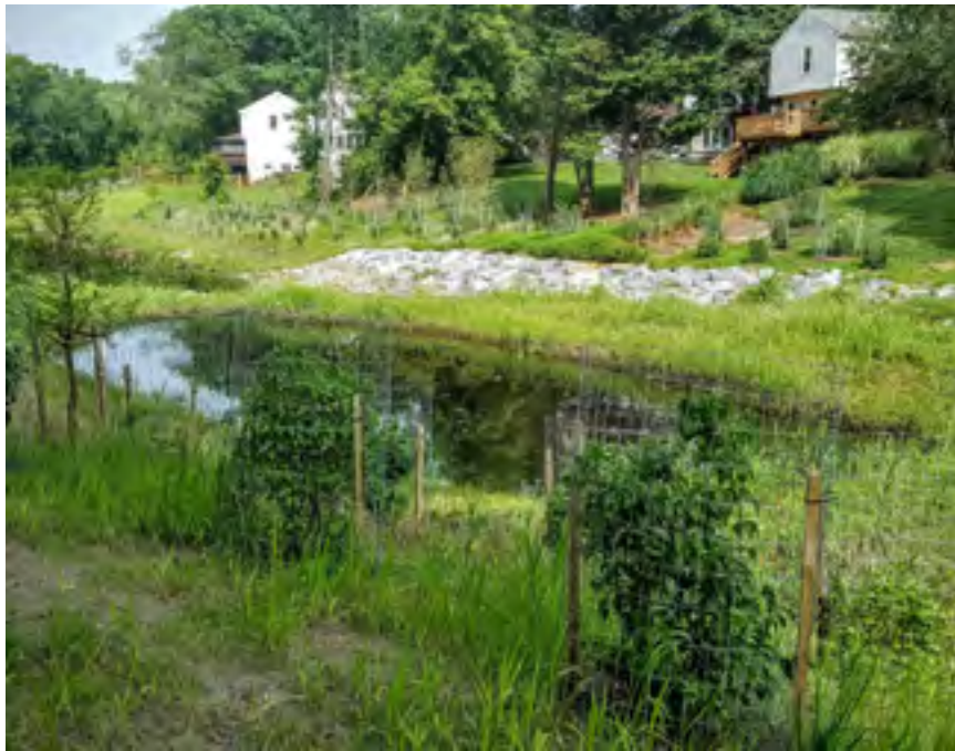
Stormwater treatment facilities include naturalized facilities such as the Horizon Hills pond, which slows and treats stormwater runoff before it enters Watts Branch Creek. This project converted a dry pond to a wet pond, meaning it retains water most of the time, which enhances water quality and provides habitat for a variety of species.
