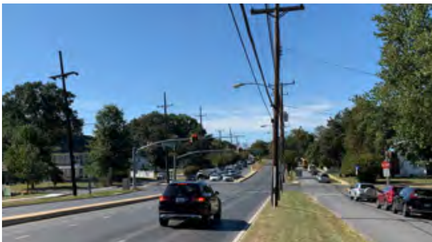
The main travel lanes and service lanes of Veirs Mill Road
