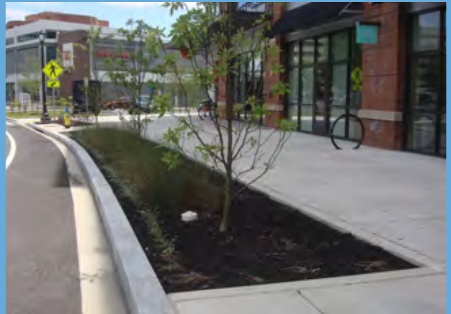
Bio-retention landscaping was installed between the sidewalk and street curb as part of new development along Dawson Avenue.
