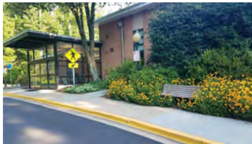
Rockville's Senior Center is an active facility dedicated to serving those who are aged 60 and older within and around the Rockville community.
