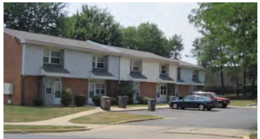
David Scull Courts comprise the majority of Rockville's public housing units with 76 total units.
