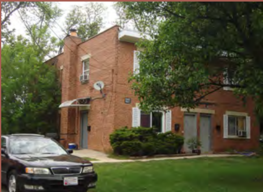
A fourplex building with four units, two above and two below, each with a separate entrance in West End, built ca. 1964.
