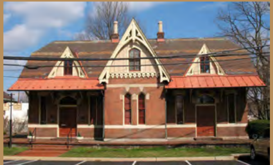
4 B & O Railroad Historic District (Designated 1974)
