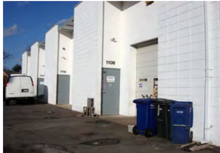
A common type of service industrial use found in the Southlawn area is characterized as 'flex space,' with a linear building divided into bays, individual addresses and entrances, and roll-up doors.
