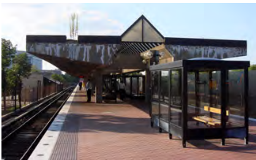
The images above show design, capacity, and maintenance issues at the Rockville transit station (from top to bottom): Buses and cars wait for traffic signals to allow an exit onto Rockville Pike (MD-355) at Church Street; Crowds queue up on the platform when escalators are under repair; Concrete spalling on the canopy is a major structural issue for the station.
