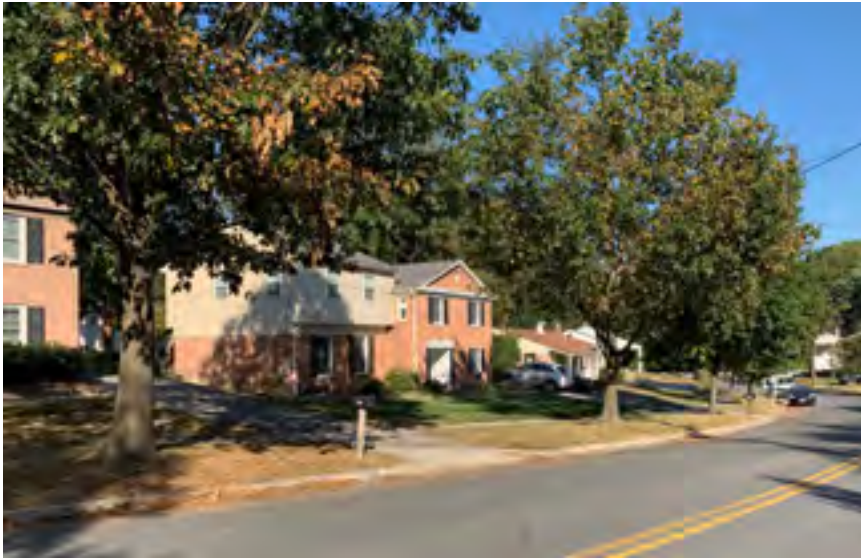
Residential homes in the planning area.
