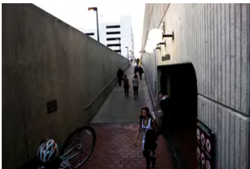
The pedestrian experience accessing the Twinbrook transit station, with its 'Brutalist' concrete forms and little vegetation, makes it unappealing. The western plaza (top) and dark ramp and stairs (bottom) lead to the station's turnstiles before rising up to the station platform by elevators or escalator.
