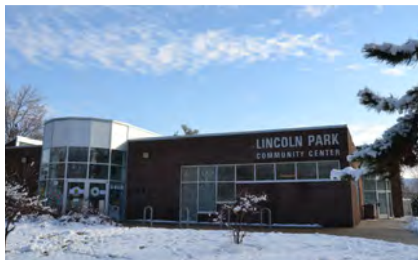
Lincoln Park Community Center is one of Rockville's most popular community facilities, providing community meeting space and after-school programs for neighborhood students.
