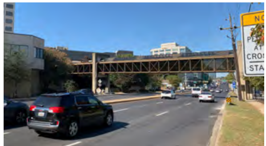
Pedestrian bridge over MD-355 connecting Rockville Transit Station to Town Center, with the former Rockville Mall building at 255 Rockville Pike beyond.
