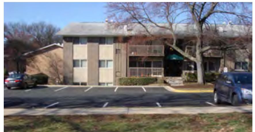
Rollins Park Apartments
