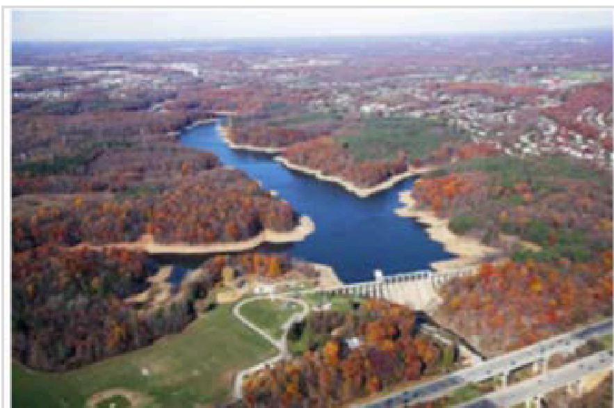
Washington Suburban Sanitary Commission's T. Howard Duckett Dam on Rocky Gorge Reservoir, Howard and Prince George's Counties
