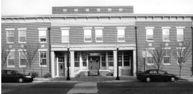
THE HIGHLANDTOWN PLAZA CO-OP IS AN ADAPTIVE REUSE PROJECT OF A FORMER STREETCAR BARN. THE FAÇADE PRESENTS A NEW FACE TO THE STREET
