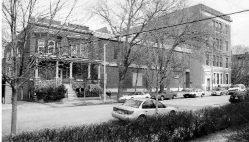
CONTEXTUAL CONSIDERATION. THE MIDDLE BUILDING WAS BUILT IN 1926, 13 YEARS AFTER THE ROWHOUSES. THE CORNICE BAND AND PORCH LINE IS CARRIED ACROSS THE NEW FACADE, RESPECTING THE PRESENCE OF THE HOUSES, BUT THE LACK OF FENESTRATION PRESENTS A BLANK FACE TO THE STREET
