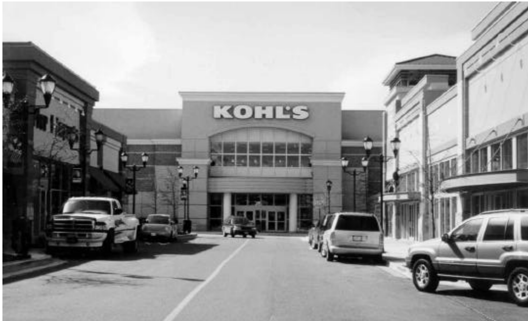
Kohl's is one of several big-box retailers located in the Washingtonian Center. Big-boxes are designed within a "main-street" environment.
