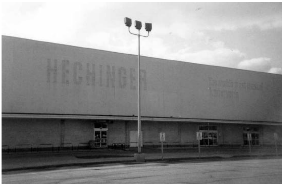
Former Hechinger store in the Reisterstown Plaza Shopping Center in northwest Baltimore, Maryland.
