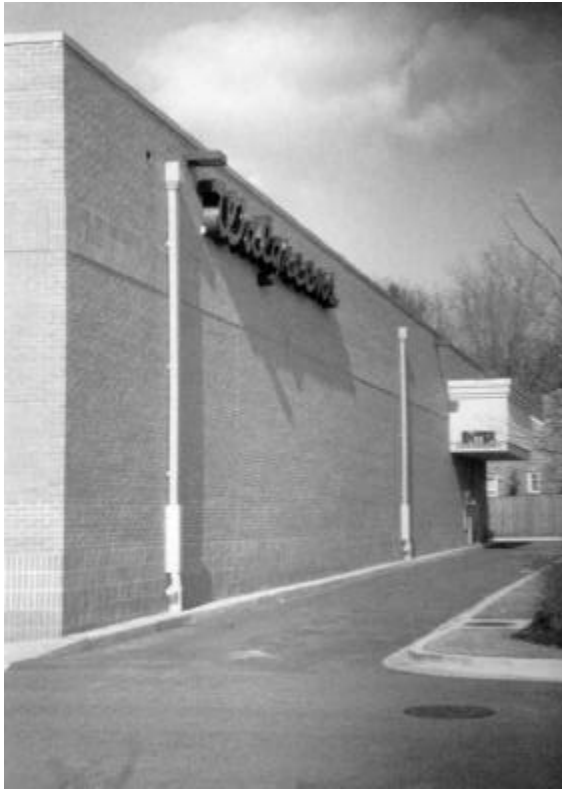
Rear drive-through prescription service at Walgreens on the corner of Liberty and Milford Mill roads.
