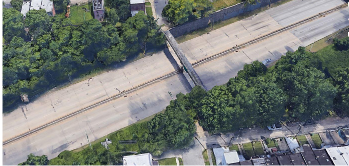
1. Pedestrian bridge (Maisel St)
