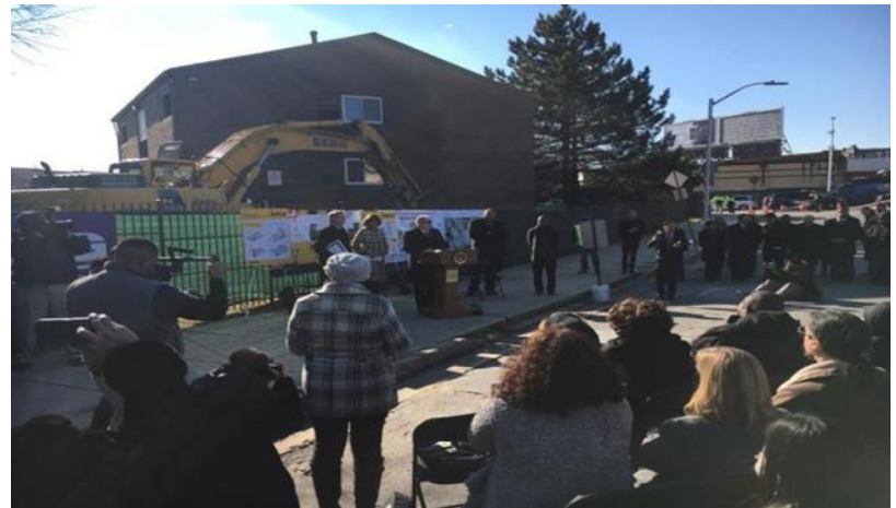
Mount Royal CDC, Innovation Village Madison Park North, $2,000,000 FY17 Award, Demolition of 202 units
