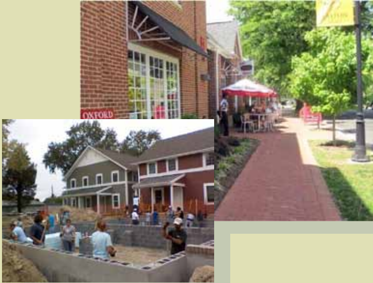
Commercial redevelopment at Dover and Aurora streets (top) and affordable residential housing built by Habitat for Humanity on Clay Street in downtown Easton.
