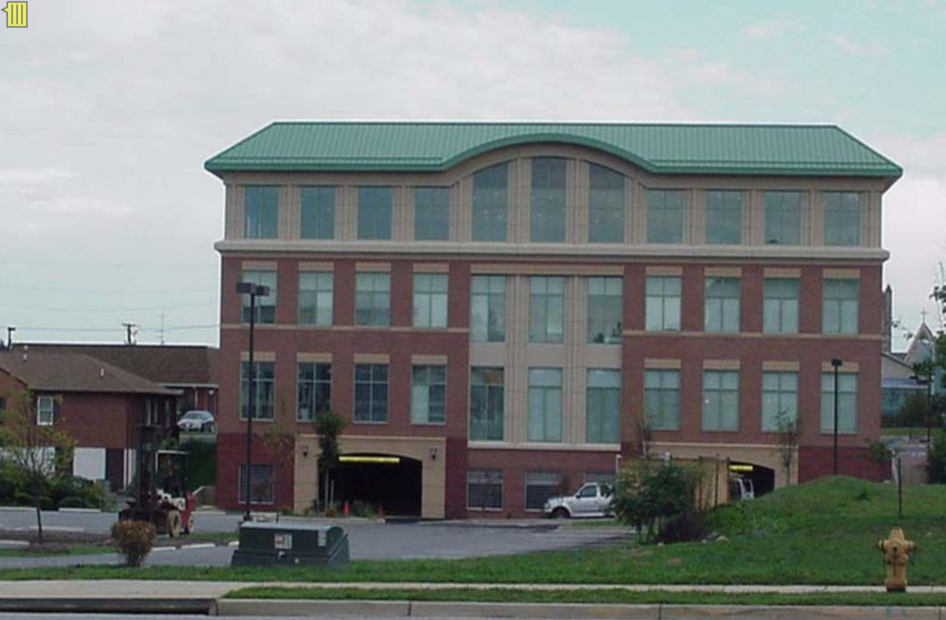
CLASS A OFFICE BUILDING IN LA PLATA
